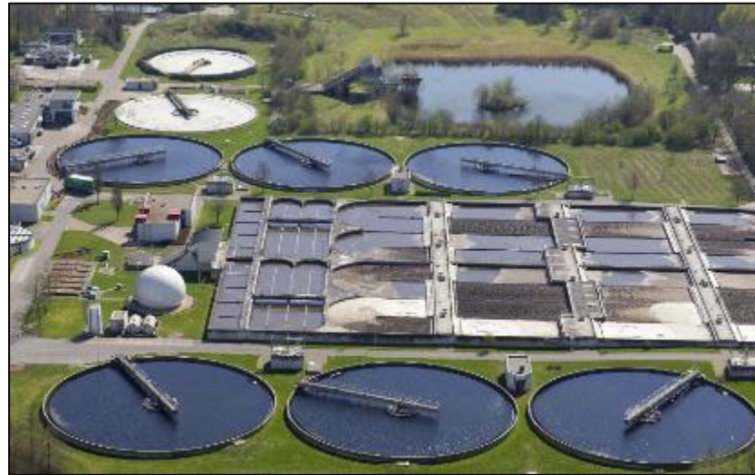
Municipal Waste Water Plant
