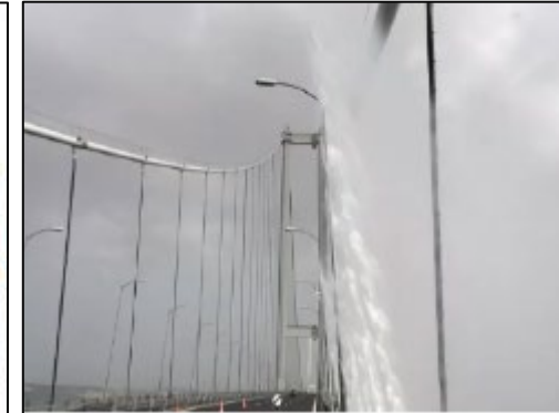
Water sprinkler system
